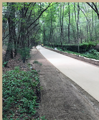
STABILIZED STONEDUST® TRUNKLINE TRAIL
